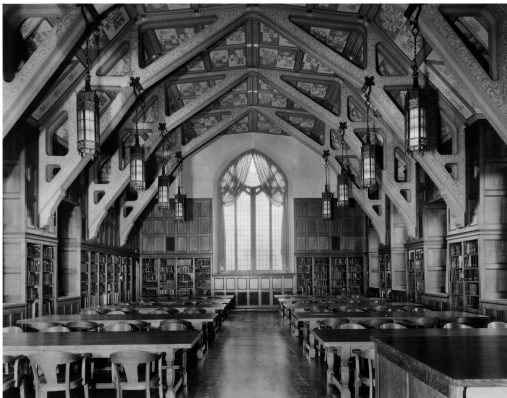
ABOVE LEFT: Figure 13. Oriental Institute Library Reading Room, ca. 1931, view to the south, showing the large rosette window (P. 19000).
